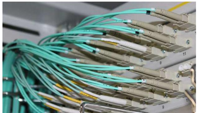
As regards the 40 and 100 Gbit/s transmission via OM3 and OM4 fibres, in the standard IEEE 802.3ba:2010 insertion losses (IL) on the transmission line of max. 1.9 dB (OM3) and 1.5 dB (OM4) inclusive of fibres are defined. Including fibres and modal noise, just 1.5 dB / 1.0 dB are left over for all connectors together. That is an acutely narrow margin in terms of practical application.
